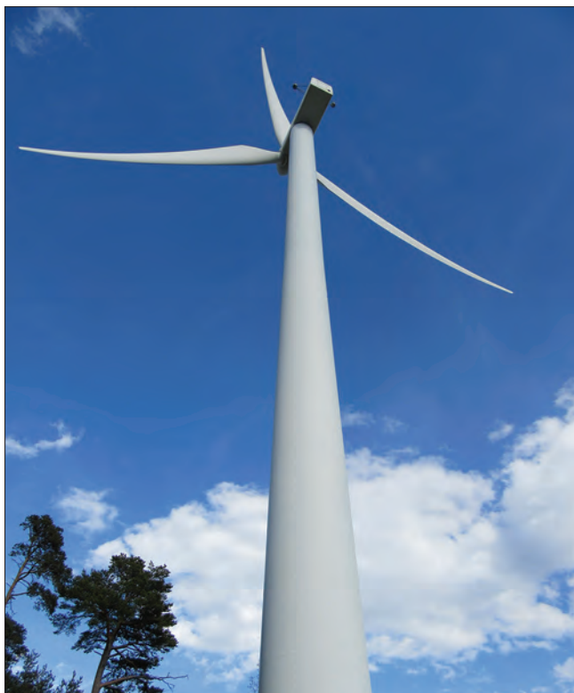
1. Saint-Denis, impianto a Puy de Saint-Évence: torre eolica. (D. Martinet)
