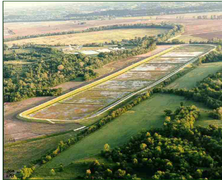
Columbia Regional Wastewater Treatment Plant (Missouri, USA)
