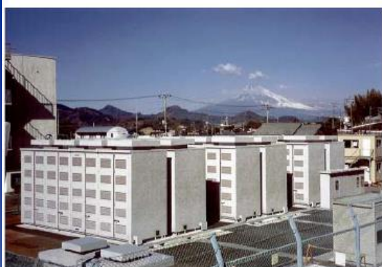
6MW / 48MWh at TEPCO's Ohito Substation
