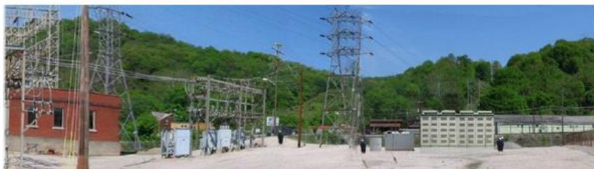
6MW / 48MWh at TEPCO's Ohito Substation
