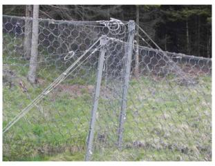
Figure 8: Flexible rockfall barriers are subject to technical standardization and approval (picture by Rudolf-Miklau)
