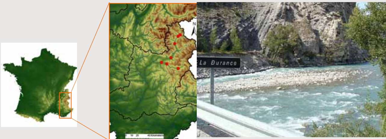
Figure 2.7: Location of seven hydrologic stations in the Upper Durance and picture of a typical torrential stretch
