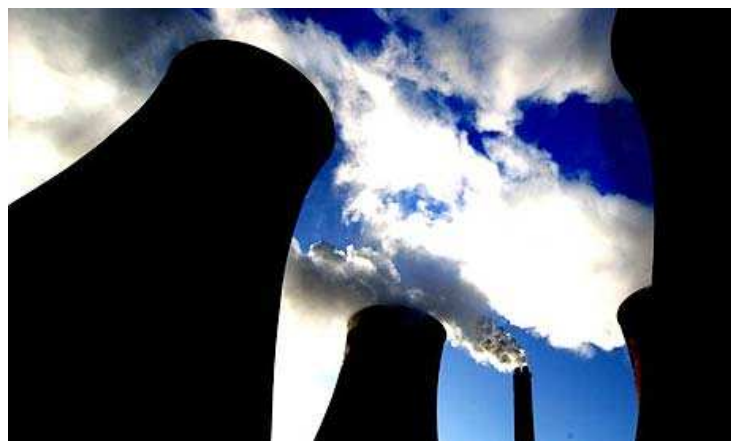
Cooling towers at Eggborough power station, near Selby. Photograph: John Giles/PA
