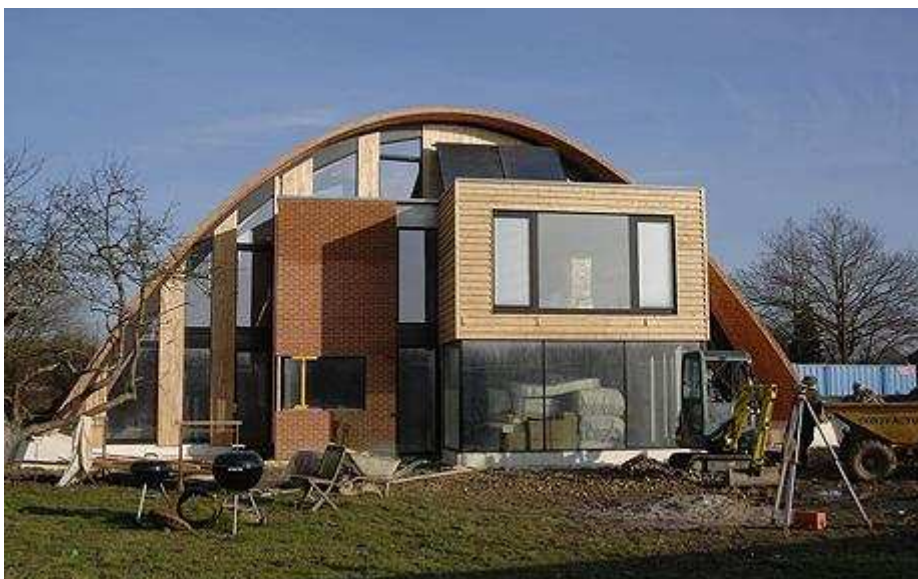
Eco-house: The unusual dome-like design is based on a Medieval technique, originating in Spain, known as 'timbrel vaulting' Photo: MASONS NEWS SERVICE
